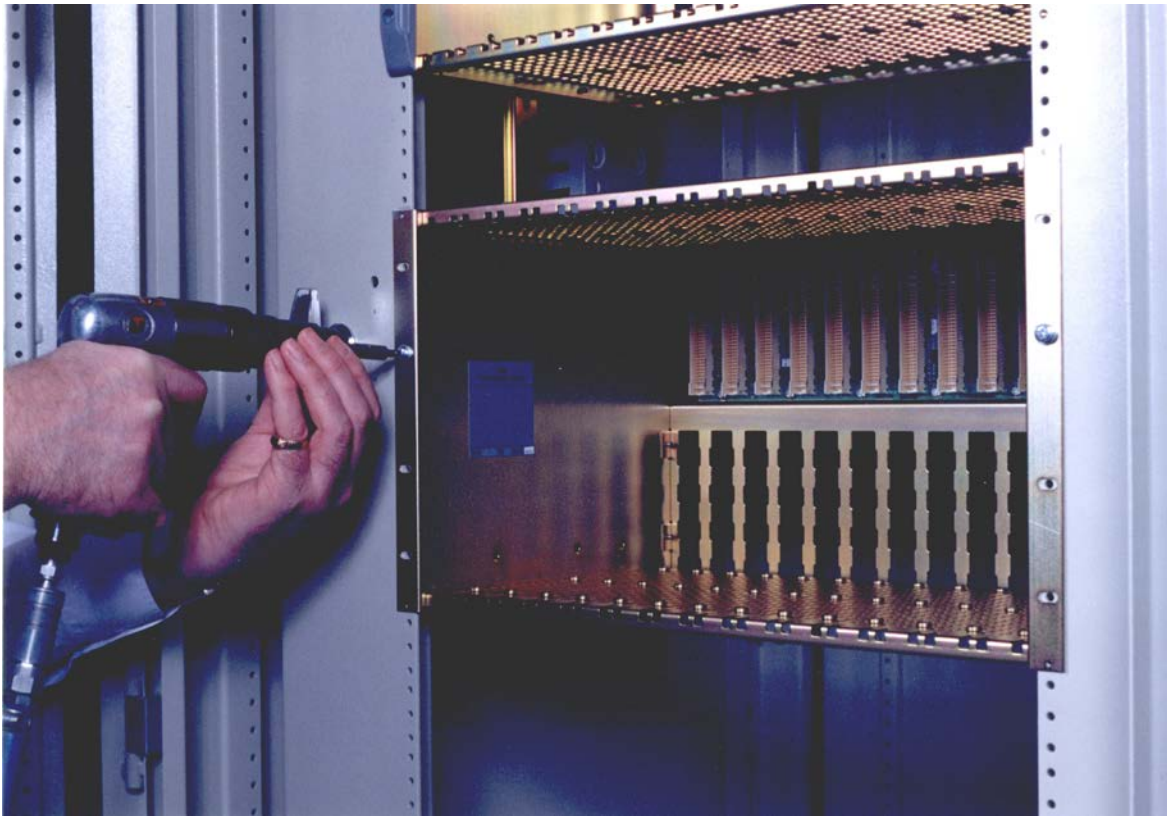
Figure 9 Installation of Chassis
